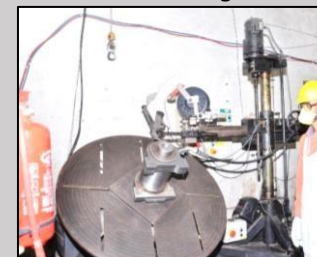
Automatic Positioner Welding
